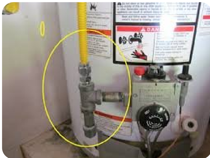
WATER HEATER IN-CORRECT WAY
